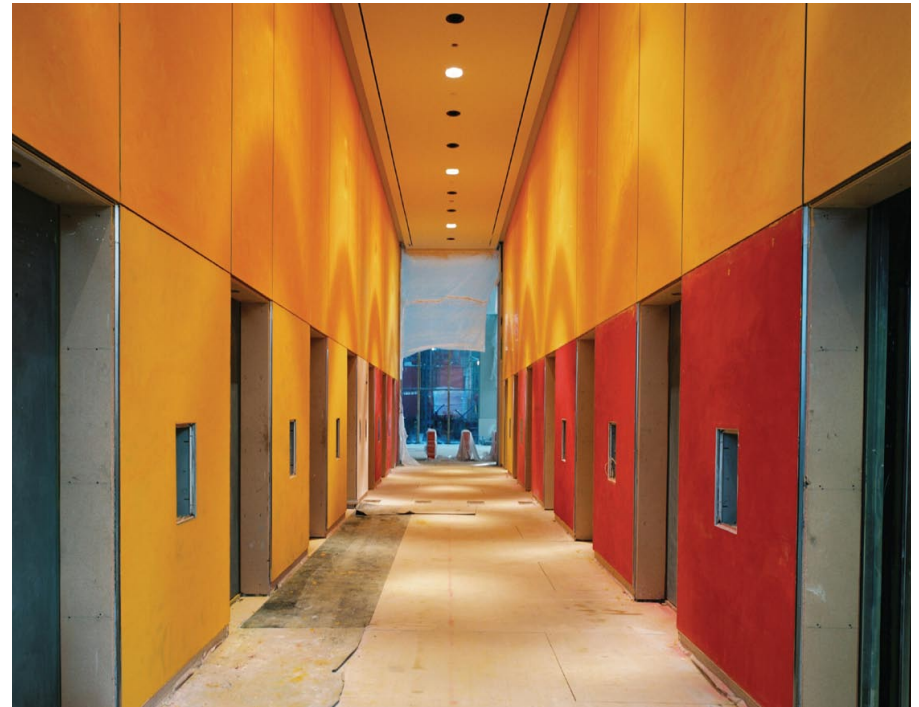
ABOVE AND OPPOSITE The key to maintaining an open and light feel within the lobby’s corridors was ringing the street fronts with all-glass facades.
